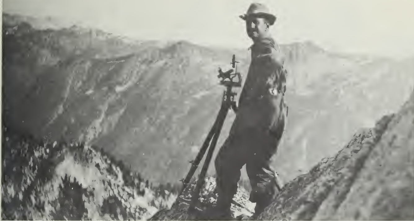
In 1914 the surveyors called this "typical mountain work in the West." The mountains are in Washington State. The instrument is a solar compass with a telescopic attachment.
