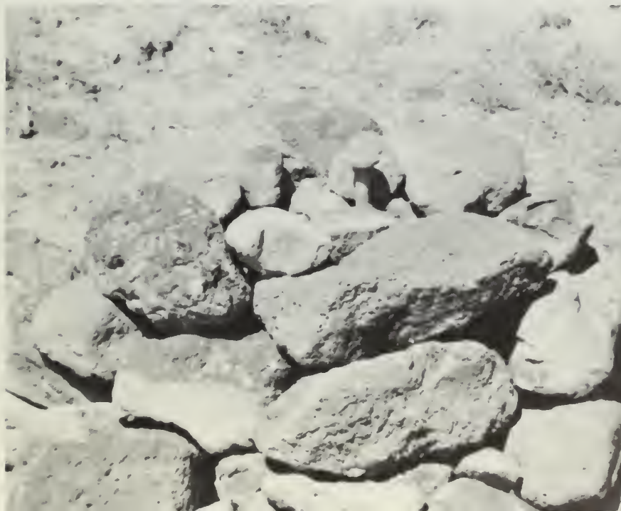
LEFT: A 1/4-section corner in T.29N., R.27E., Mt. Diablo Meridian, near Cottonwood Springs, west of the Seven Troughs Mountains in Nevada. There are thousands of similar corners in the United States. (70)
