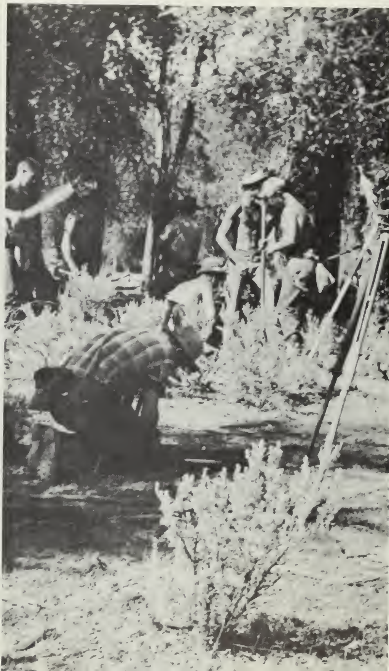
August 26, 1948. Utah-Wyoming State line near mile post 37. The survey party is under the direction of F. Wayne Forrest. The man in the foreground (kneeling) is stamping the section number into the brass cap of a survey monument.
