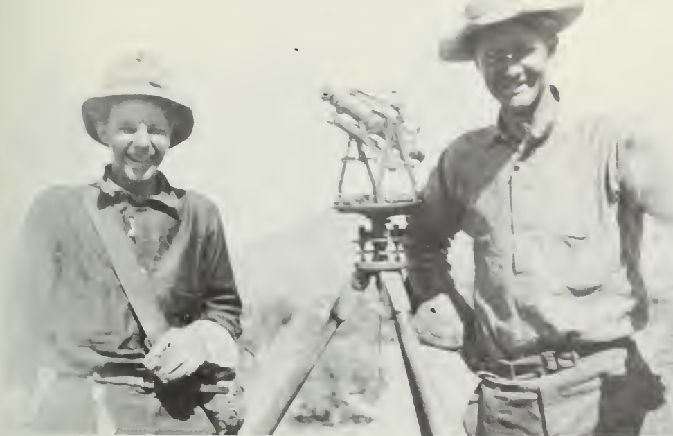
Hopi Indian Reservation, Arizona, 1910. Left to right: Van and T.Y. (called Ty) White. The instrument is a Gurley with a Burt Solar Attachment.
