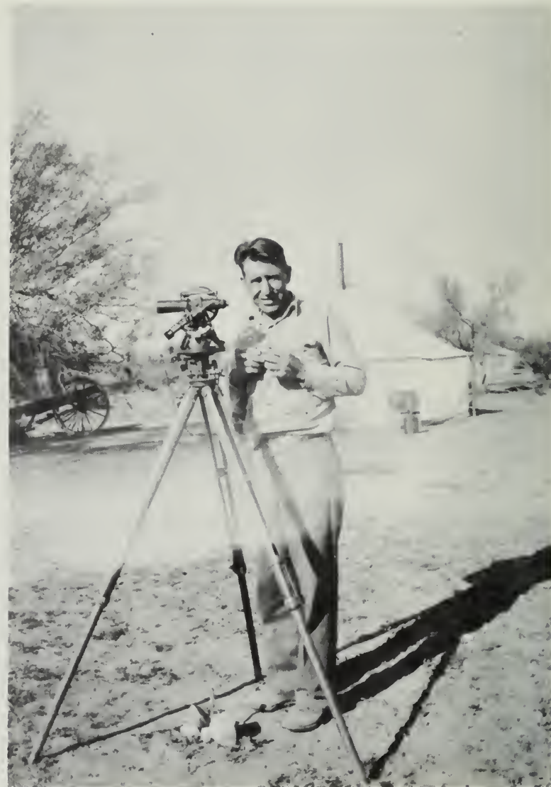
Elliot Pearson at camp at Gila Bend, Arizona, 1947. The instrument is a Hellgate model Gurley transit. (70)
